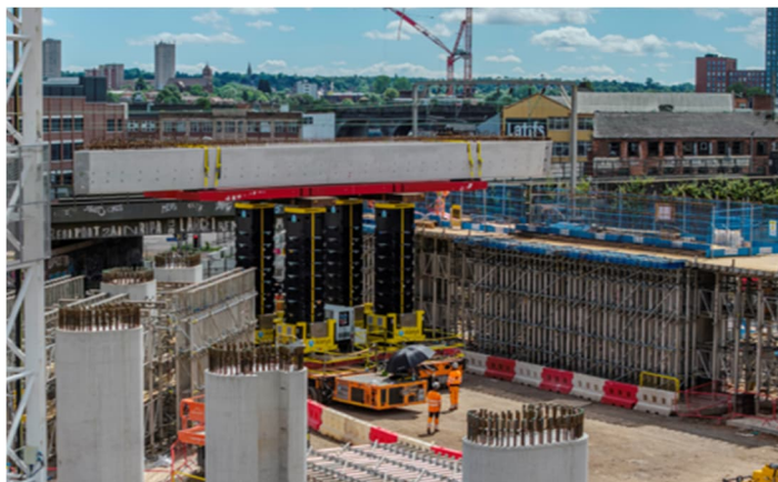
First beams lifted for Birmingham's Curzon Street station
